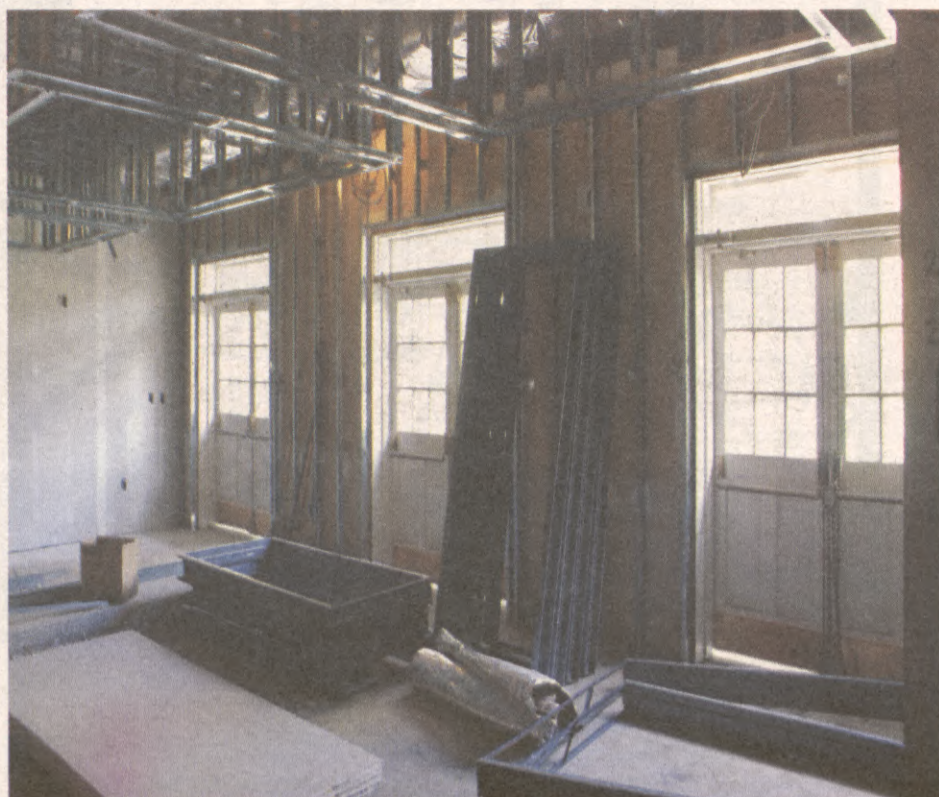
Second floor lobby of McClurkan, with original doors.
