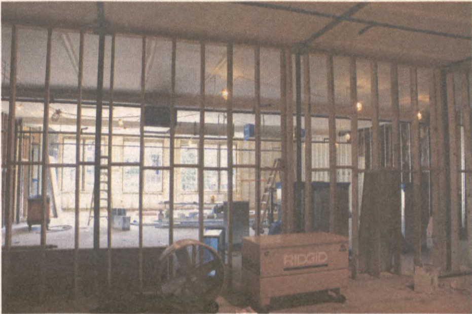
Second floor classroom behind auditorium in McClurkan.
