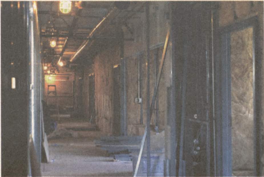
New third floor hallway of McClurkan.
