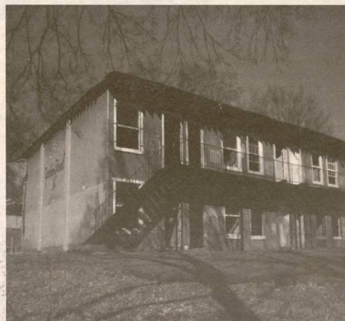
The Castanea Community Center at 12 Garden Street. (photo by Jordan Taylor)
