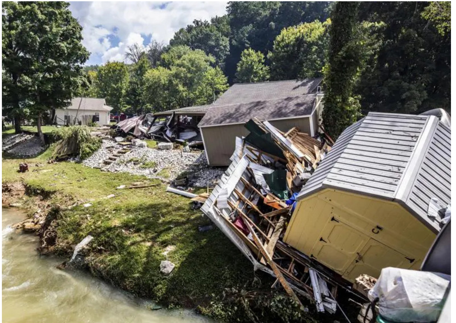
Flood damage along Trace Creek in Waverly. Photo courtesy of The Associated Press
