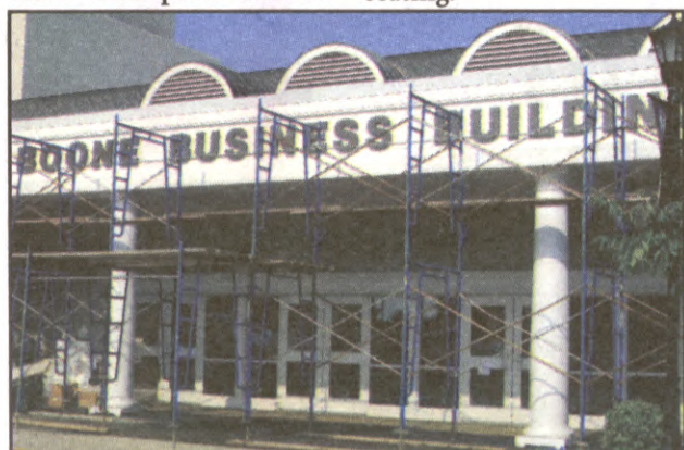
Boone Business Building during summer renovations. (Photo courtesy of Trevecca Marketing Department)
