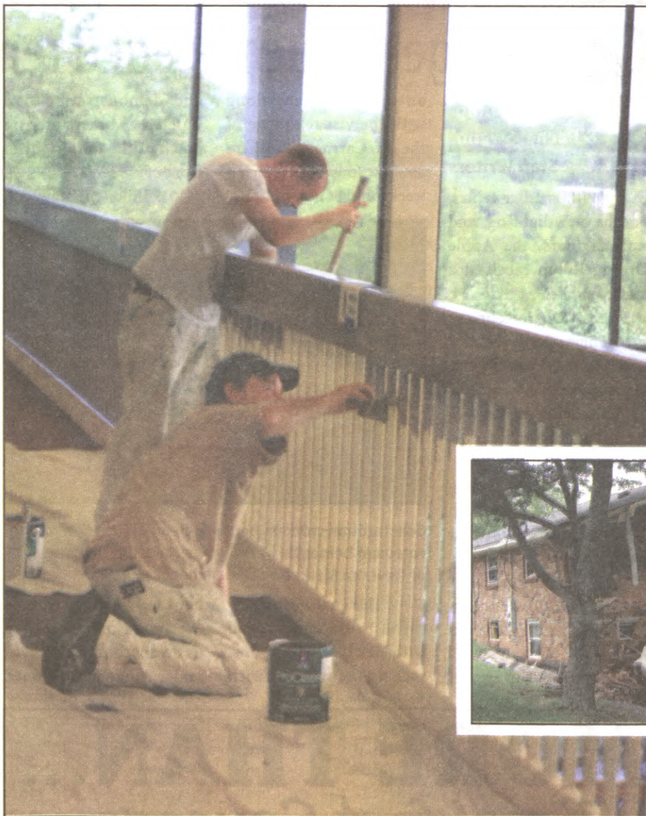
Workers paint the railing on third floor of Jernigan Student Center. (Photo courtesy of Trevecca Marketing Department)
