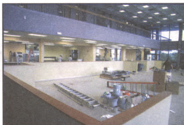
Construction workers begin to clean up the newly renovated caf before the new tile was laid. (Photo courtesy of Trevecca Marketing Department)
