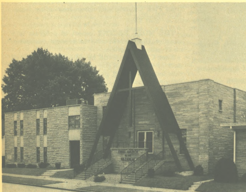
REV. GEORGE SCUTT , superintendent of the Northwest Indiana District, preached the dedicatory message on the occasion of the completion of a $45,000 building and remodeling project of the Crawfordsville (Indiana) First Church. A two-story educational unit was completed and the sanctuary refurbished, according to Pastor W. S. Muir.
