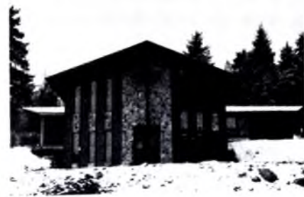
The Sitka, Alaska, church was host November 16 to General Superintendent Orville W. Jenkins at a day of dedication for the recently completed two-story educational building and remodeled sanctuary. The building was completed during the pastorate of Rev. Al Haynes, presently of Anchorage, Alaska, Hillcrest Church. Rev. and Mrs. Haynes were special guests for the day, along with District Superintendent Robert W. Sheppard. Rev. Glen L. Van Dyne is the present pastor.
